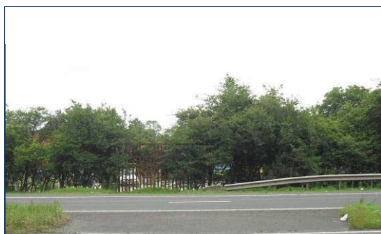
③ Steel fence at A1 southbound carriageway
