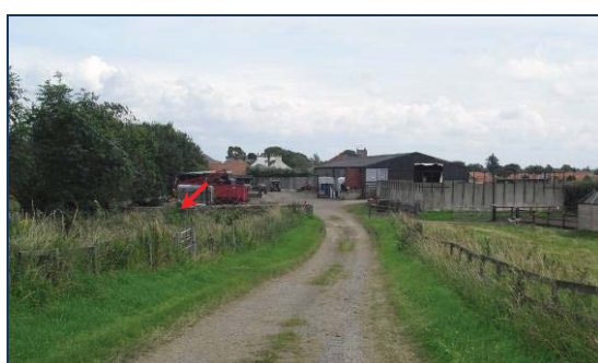
④ Gated access to/from bridge eastern approach track
