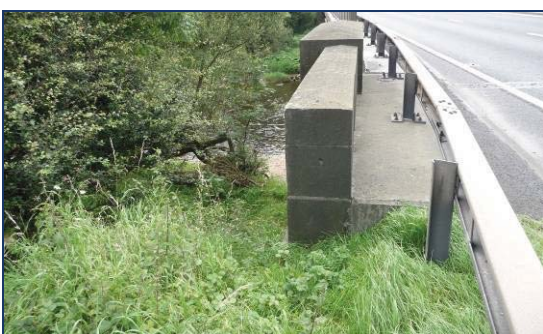
④ Embankment down onto PROW from A1 above
