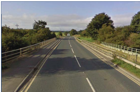
① A6136 Catterick Road overbridge
