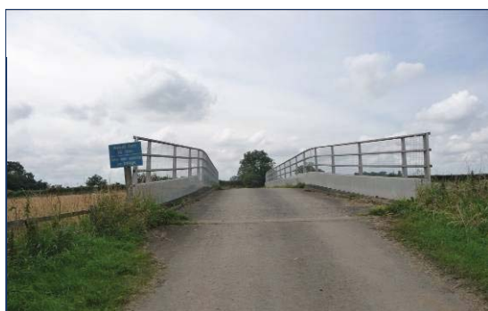
③ Accommodation overbridge at Manor House Farm
