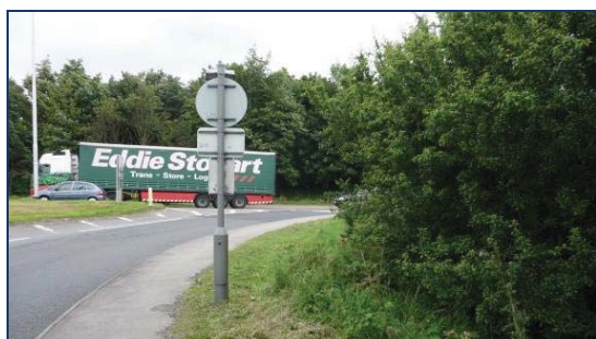
② Restricted visibility over A6108 exit arm
