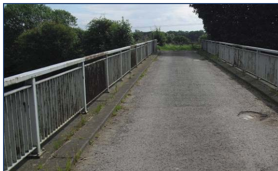
② Accommodation overbridge
