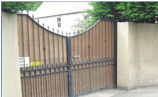
① Gates preventing access onto route at Oak Grange
