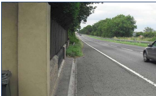
② Northbound carriageway north of access location
