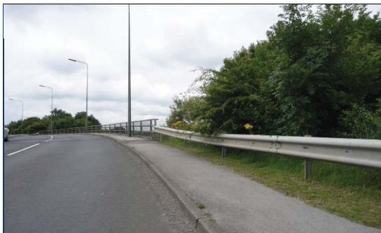
① Footway's eastern approach to overbridge
