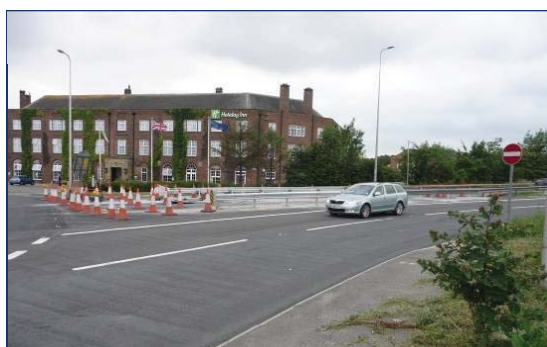
③ Absence of crossings over A66 entry/exit arms
