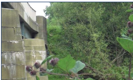
② Bridge carrying A1 over River Swale (eastern face)
