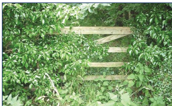
④ Gated access at A1 boundary
